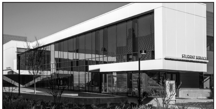
The new Student Services and Administration buildings will serve more than 11,000 students each semester and are the welcoming "front door" to the Santa Maria campus.
