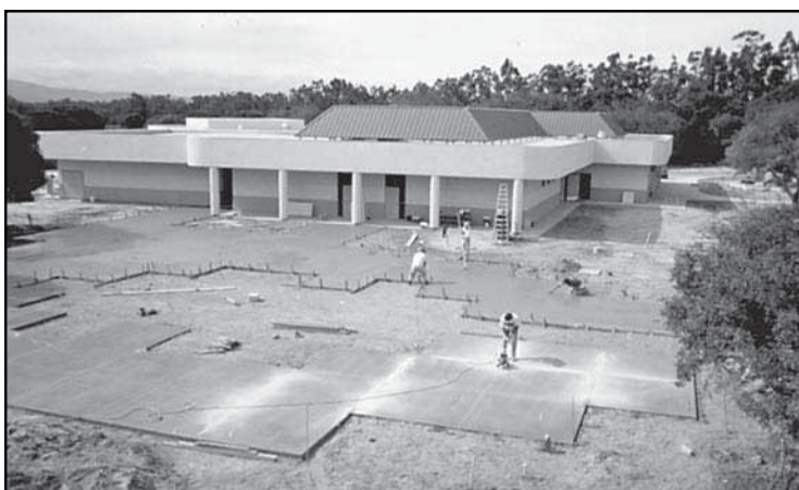
Lompoc Valley Center: Construction of the quad area, circa 1998
