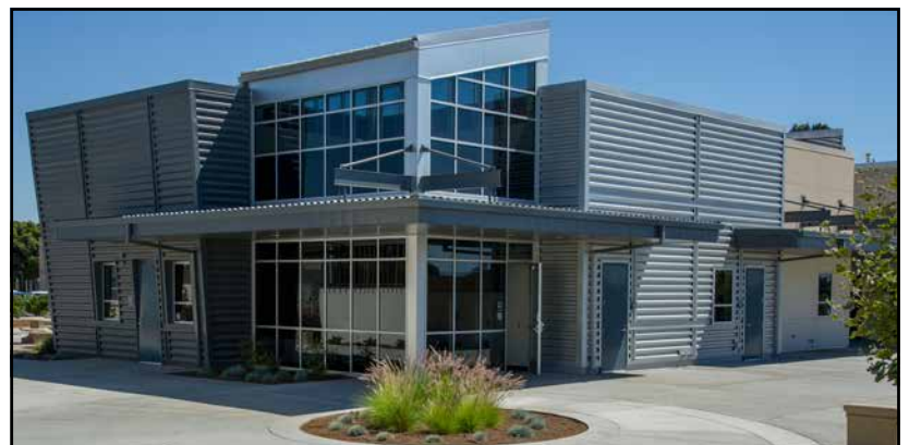
The Industrial Technology Complex was completed late fall 2013 and provides new and expanded facilities with space for the IT programs including: automotive transportation technology, auto body technology, architecture/engineering technology, machine technology, welding, and administrative support.
